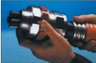
2. Install StarTeck XP™ on cable
