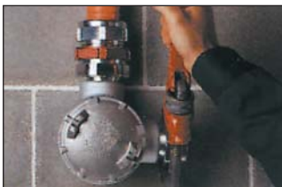
5. Install hub on enclosure
