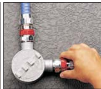
7. Insert cable and tighten red union
