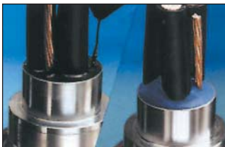
4. Pot cable (using liquid or putty)
