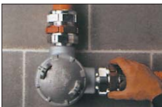
6. Insert cable and tighten red union
