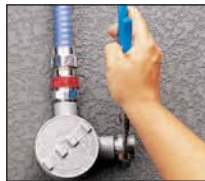
6. Insert hub on enclosure
