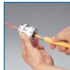
Install TCAX fitting on cable
